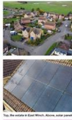
Top, the estate in East Winch. Above, solar panels.
